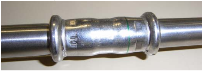
Figure 2: (before test start) Test sample 1, 611793.6S - pipe 1.4401 Ø22
